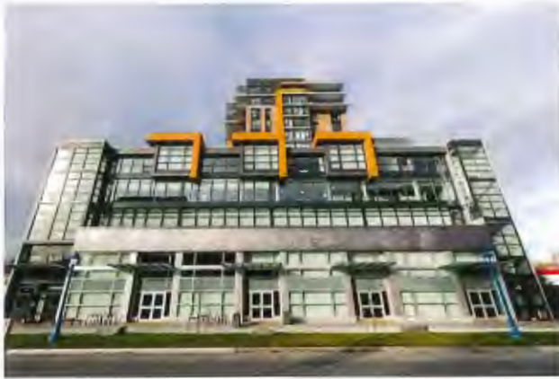
Storeys Affordable Housing Development
