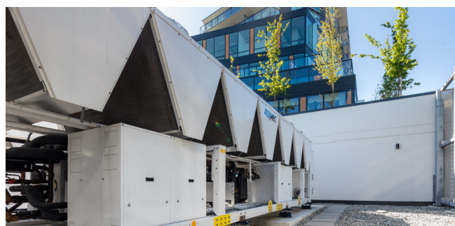
CCDEU Expansion Project
