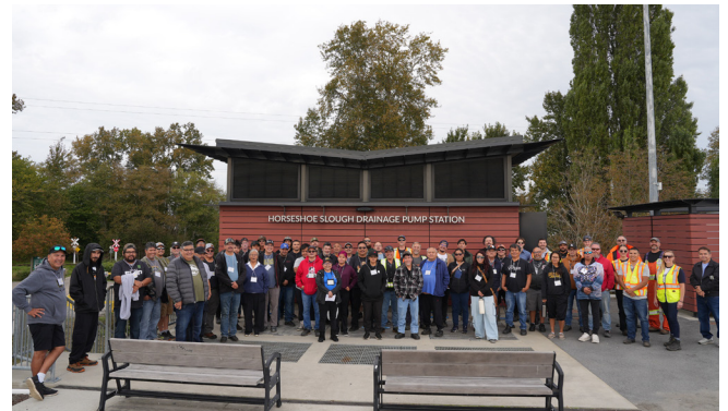
Horseshoe Slough Drainage Pump Station
