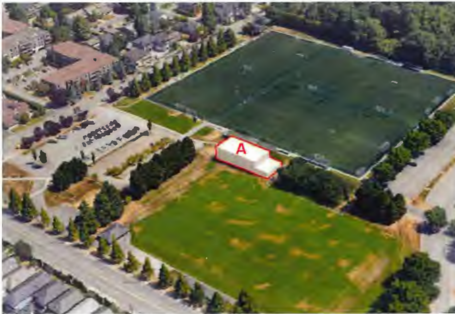
Figure 1: Site A – Aerial View from Northeast
