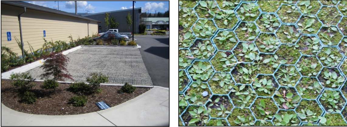
Figure 12-2: Example of reinforced clean crushed gravel and Geogrid
