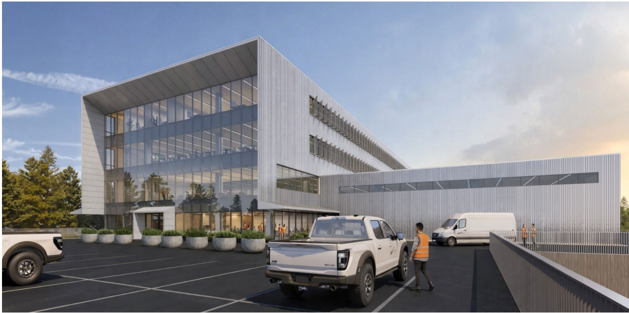
Northwest View – From Fleet Parking on Level 1
