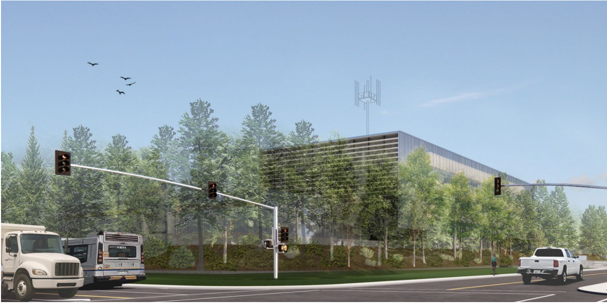
Southeast View – From Lynas Lane and Westminster Highway Intersection
