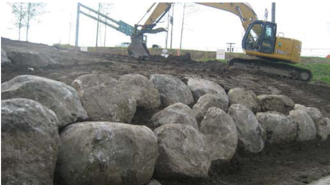
INSPIRATION: Boulder edge under construction
