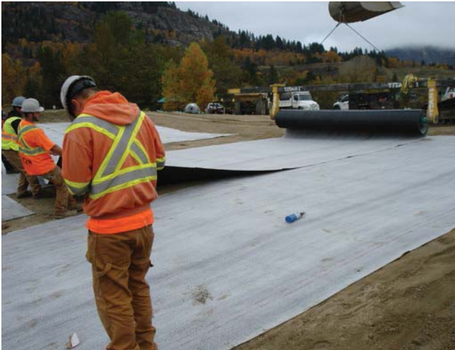
EXAMPLE: Clay set between geotextile layers installed over protective sand cushion.
