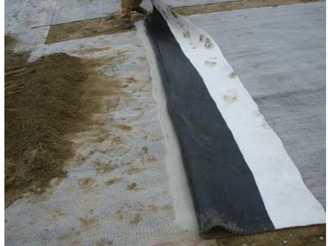
EXAMPLE: Bentonite applied to seal lap joints.
