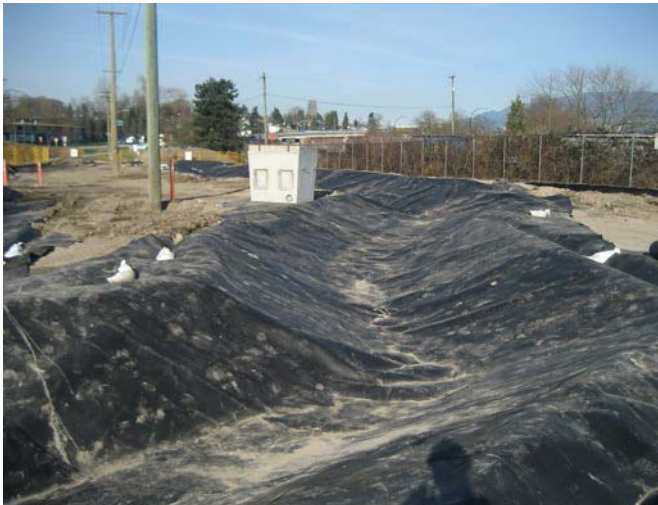
EXAMPLE: Installation of HDPE liner in creek channel.
