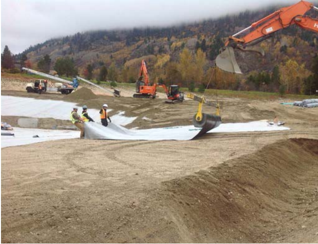
EXAMPLE: Bentonite liner being rolled out.
