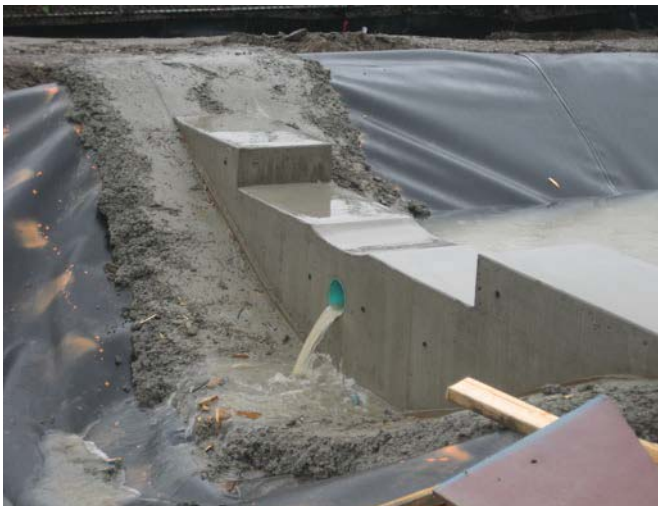
EXAMPLE: Weir structure for pond transition.
