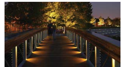
INSPIRATION: The major canal crossings should incorporate decorative railings, high quality materials, and lighting.
