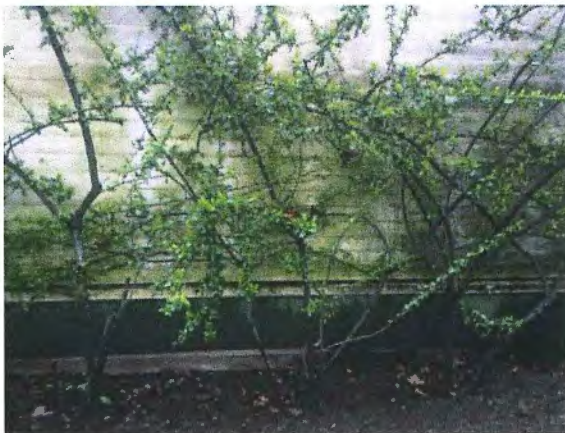
Figure 26 – Vegetation in close proximity to the exterior wall and staining on the cladding.
