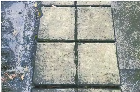
Figure 72 – Debris between roof pavers and obstructed drainage.
