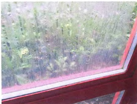
Figure 33 – Failed IGU.
