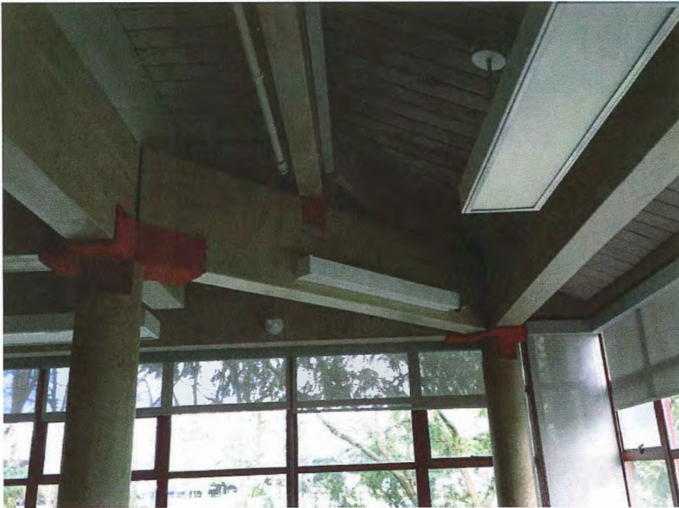
Picture 1 - Exposed Timber Roof Framing
