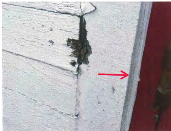
Figure 35 – Failed sealant around window.
