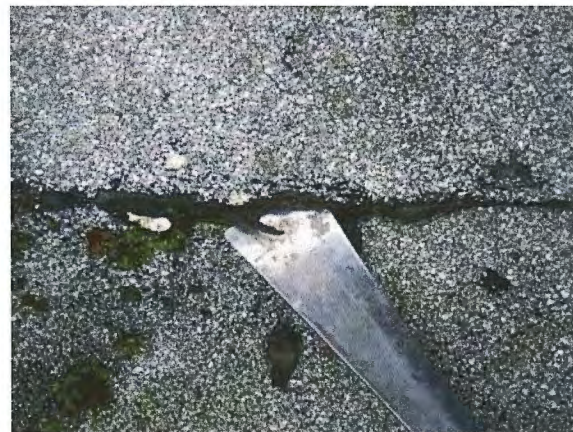
Figure 66 – Failed roofing membrane seams.
