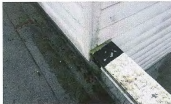
Figure 76 – Suspect saddle interface and exposed self-adhered membrane.
