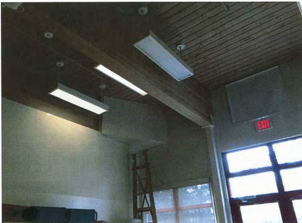
Picture 2 - Glulam Beams Clearspan Activity Room
