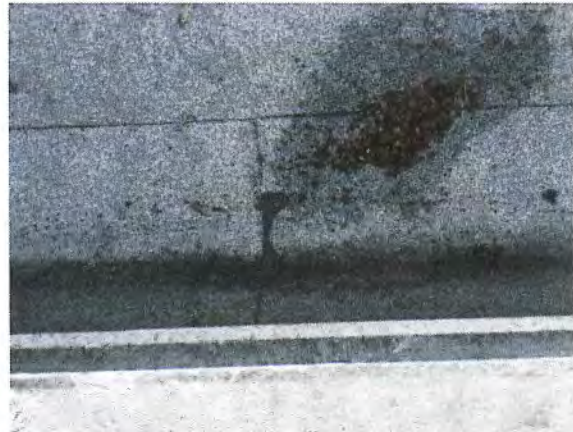
Figure 64 – Roofing membrane bleed out.
