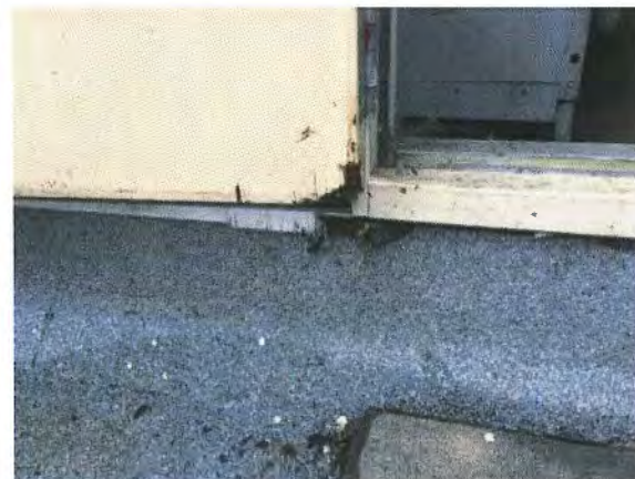
Figure 68 – The roofing membrane not extending into door rough opening and has exposed edge.
