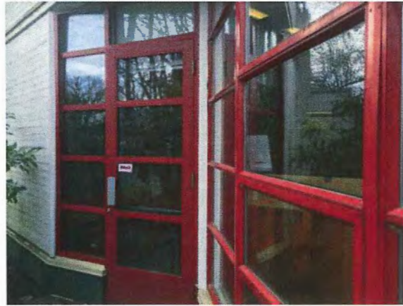
Figure 30 – Aluminum-framed storefront window.
