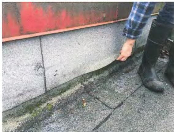
Figure 65 – Roofing membrane not well adhered.
