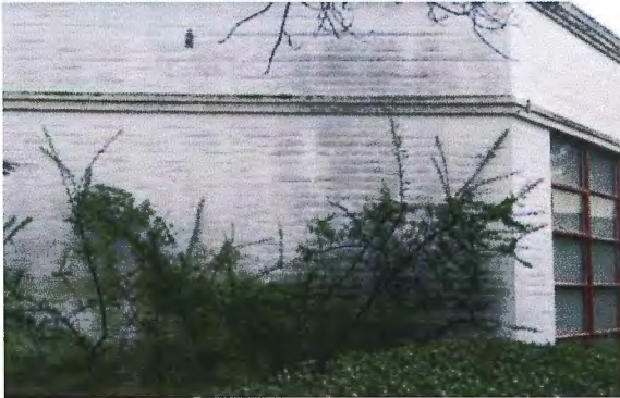
Figure 19 – Stained horizontal cedar siding.
