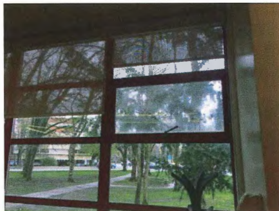
Figure 31 – Casement opening vent.
