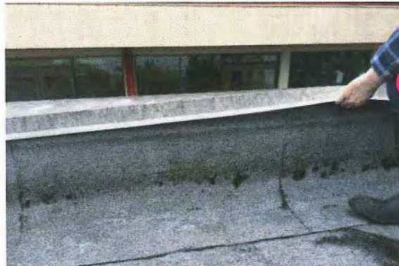
Figure 74 – Roof parapet metal flashing not well-secured.
