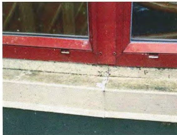
Figure 56 – Metal flashing seam unsealed and only overlapped.
