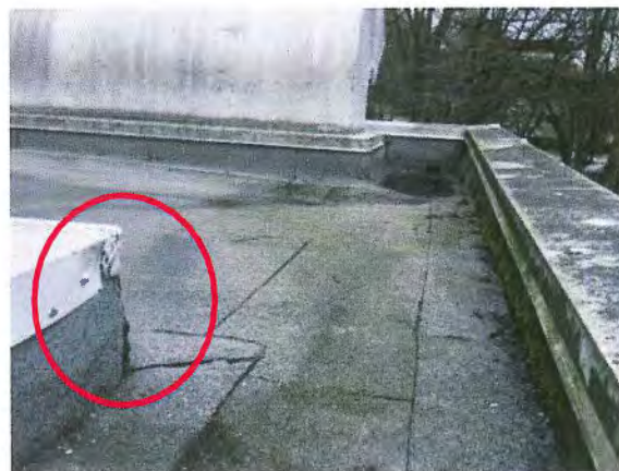
Figure 67 – Metal flashing cutting into the roofing membrane.
