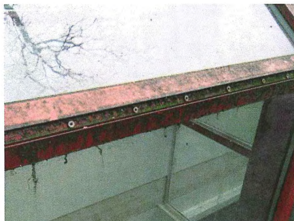
Figure 50 – Corroding fasteners at skylight (typical).
