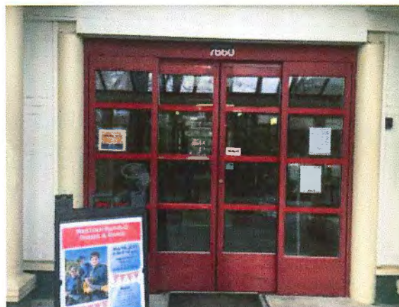
Figure 39 – Glazed automatic sliding door.
