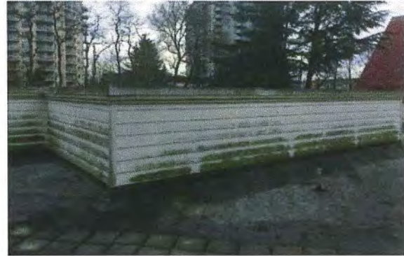
Figure 20 – Stained cementitious horizontal siding at the roof.
