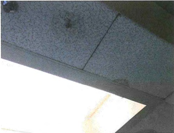
Figure 51 – Signs of water ingress at skylight.
