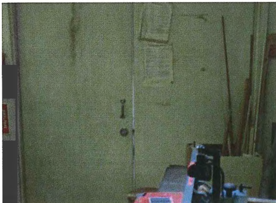
Figure 46 – No gasket around the door and daylight is visible through the door slabs.
