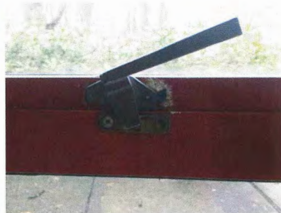
Figure 32 – Broken window hardware.
