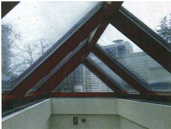
Figure 48 – Pressure-plate aluminum glass skylight.
