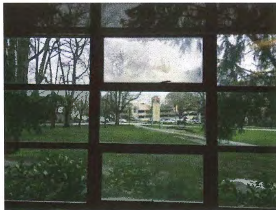
Figure 34 – Failed IGUs
