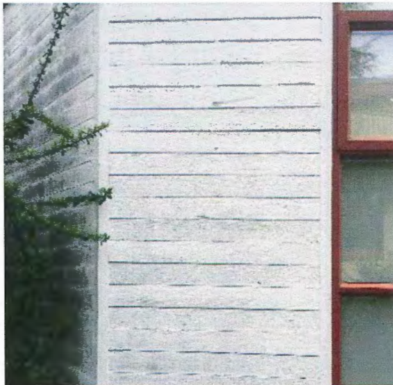
Figure 8 – Painted horizontal cedar siding
