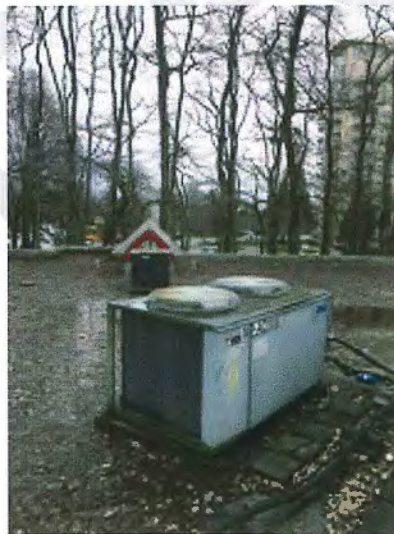
Figure 3 – Existing outdoor Split Condensing
