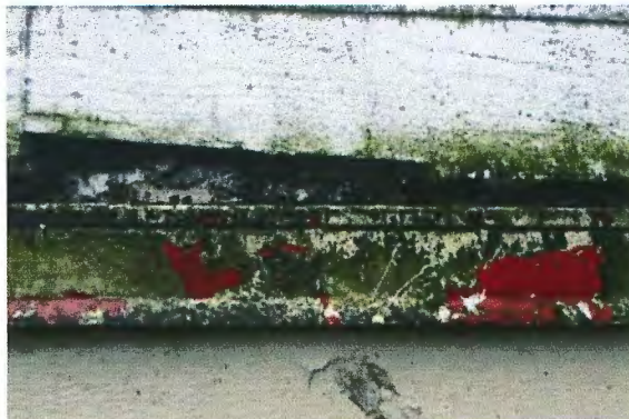
Figure 17 – Delaminating paint on metal flashing.
