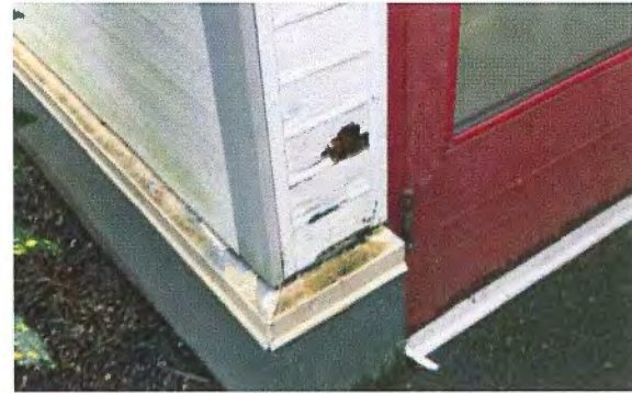
Figure 22 – Deteriorated horizontal cedar siding.
