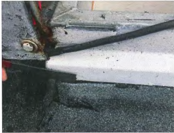
Figure 69 – Exposed edge of roofing membrane.
