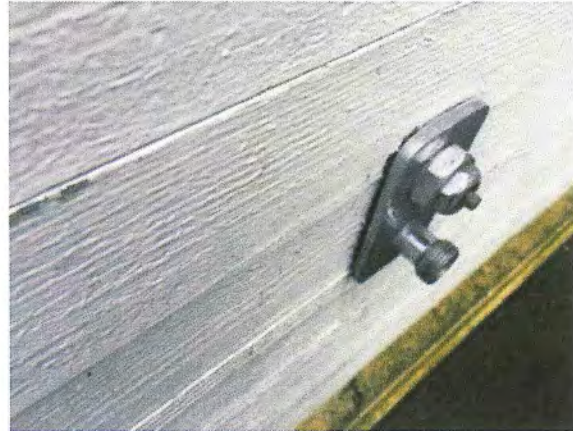
Figure 55 – Wall penetration (typical).
