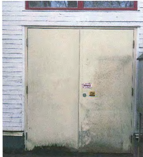
Figure 38 – Pressed steel door.
