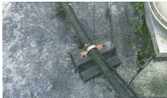
Figure 82 – Corroded fasteners at electrical cables.
