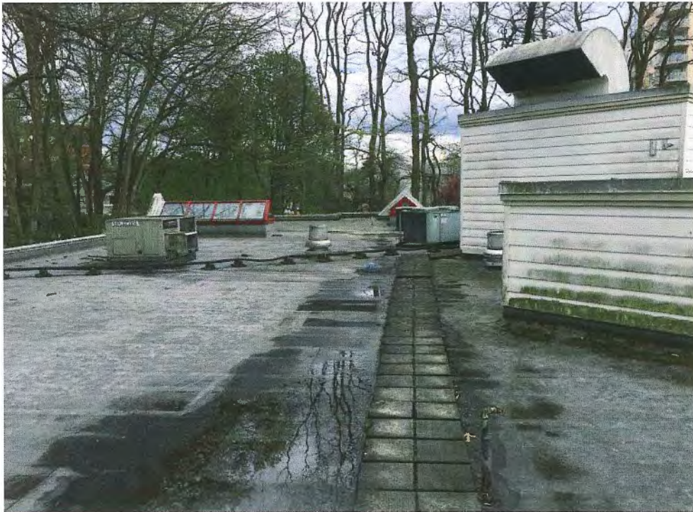
Picture 3 - Roof in Fair Condition – Drains Well. There are several Rooftop Units.
