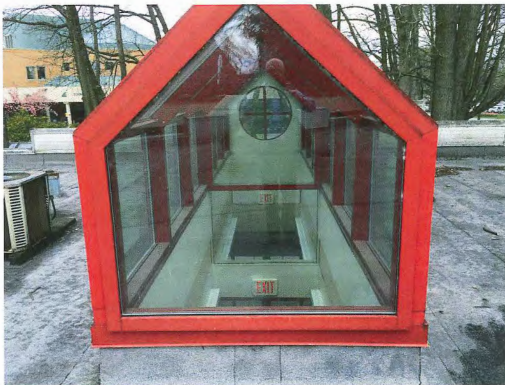
Picture 4 - Aluminum Framed Skylights
