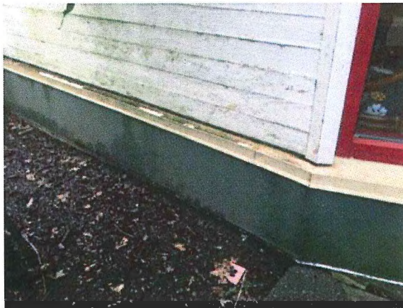
Figure 10 – Typical base of wall finished grade near the top of the slab on grade.
