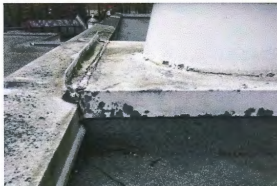
Figure 75 – Delaminating paint at metal flashing.
