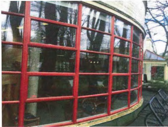
Figure 29 – Aluminum-framed windows with rolled-in glazing stops.
