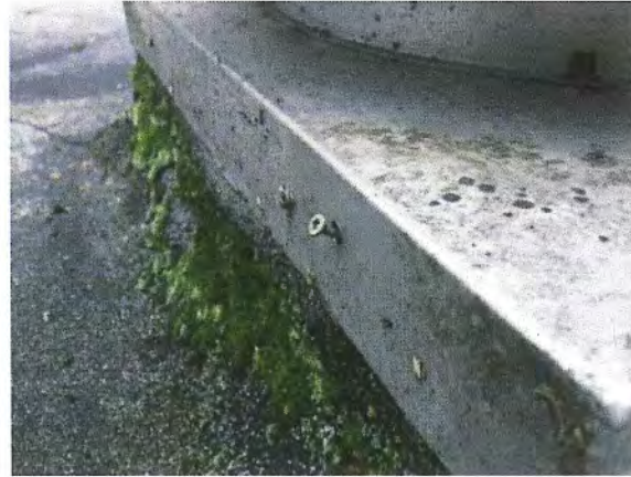
Figure 78 – Unsealed fasteners at extraction fan.
