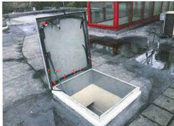
Figure 80 – Roof access hatch.
