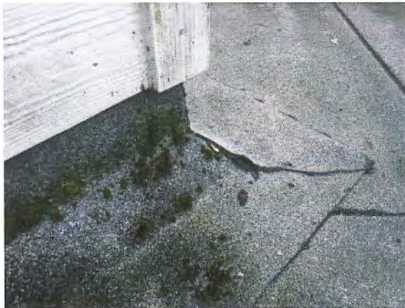
Figure 63 – Fish mouth in the roofing membrane.
