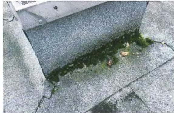
Figure 73 – Moss growth on the roofing membrane (typical).
