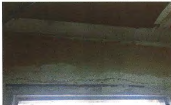
Figure 41 – Water ingress at mechanical room door head.
