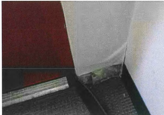
Figure 45 – Water ingress at door sill.
