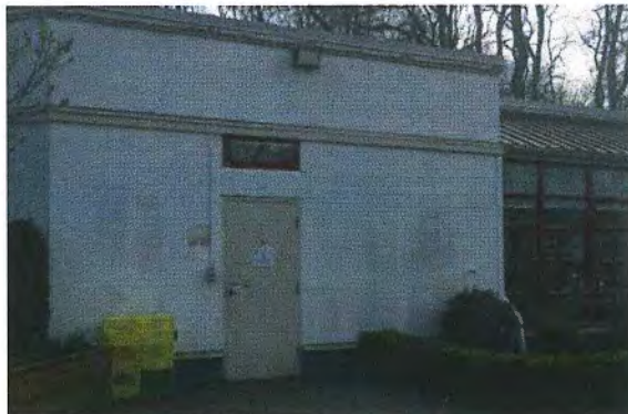
Figure 42 – Exposed pressed steel door.
