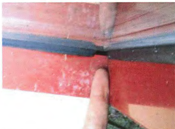
Figure 36 – Shrunken gasket at a window.
