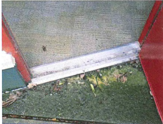
Figure 44 – Corroding fasteners at door threshold (typical).
