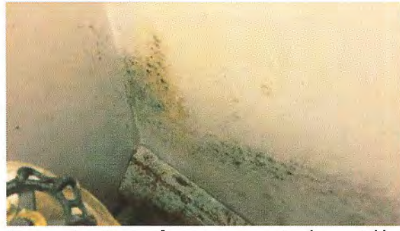
Figure 14 – Signs of water ingress in the sprinkler room, below the glass canopy to wall interface on the north-east elevation.
