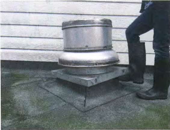
Figure 77 – Extraction fan not well secured
