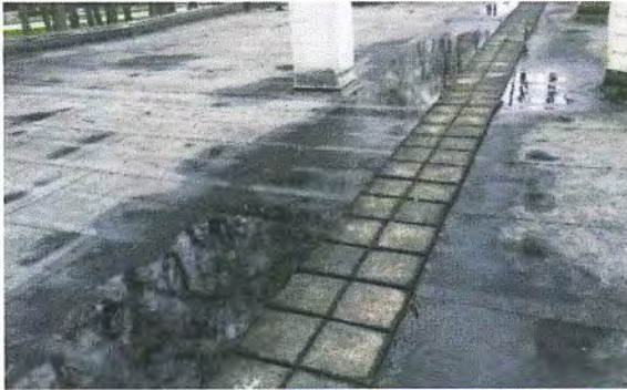
Figure 70 – Ponding water within the field of roof where pavers are obstructing drainage.
