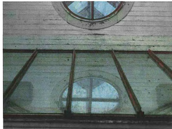
Figure 49 – T-bar aluminum-framed glass canopy.
