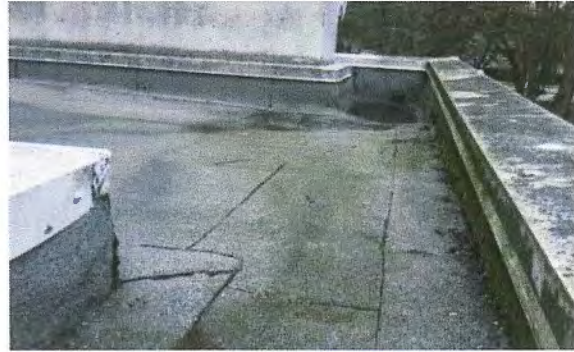
Figure 71 – Ponding water adjacent to scupper drain.
