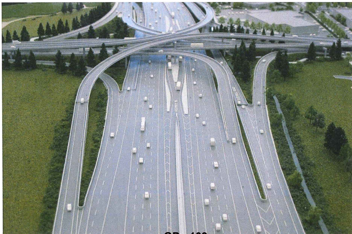
Facing south toward Steveston Highway Interchange
