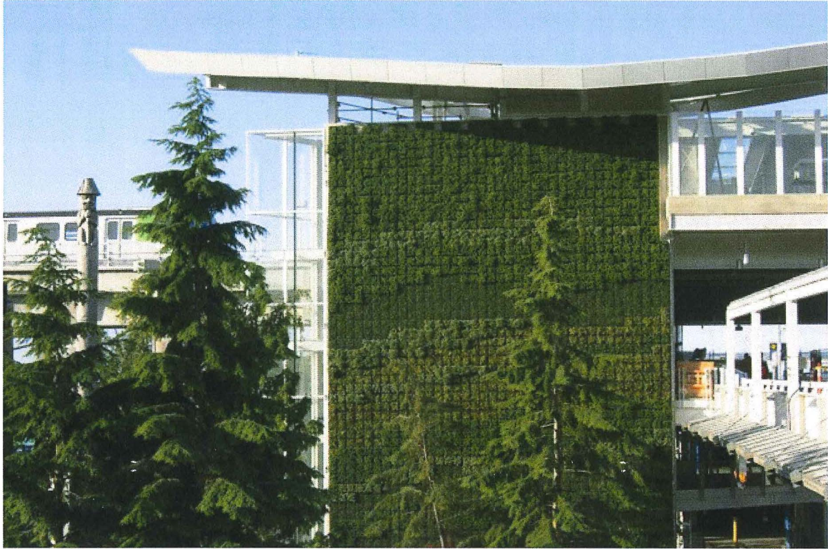
Green Wall at Vancouver International Airport [Source: Connect Landscape Architecture Inc., Vancouver, BC]
