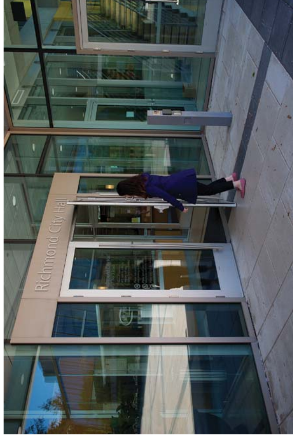
Extensive glazing at doorways into interior lobbies enhances wayfinding and building security. Install security hardware with ease of use and accessibility in mind.
