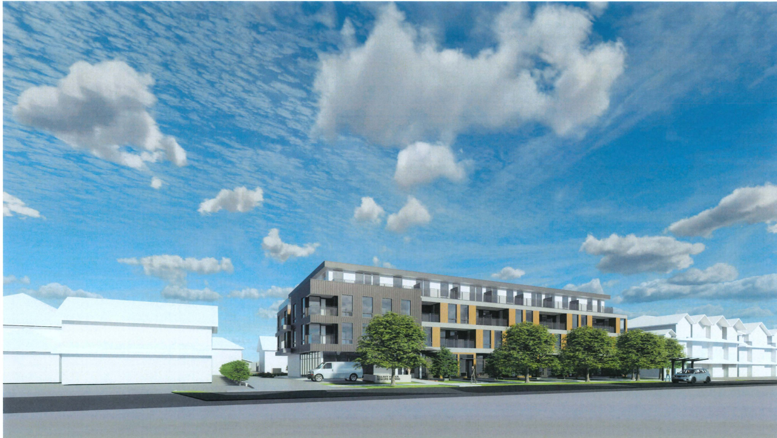
VIEW FROM THE SIDEWALK
