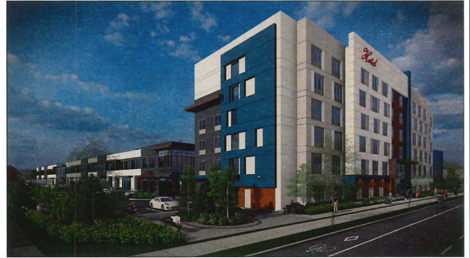
2 VIEW OF SOUTHWEST CORNER SCALE: N.T.S.
