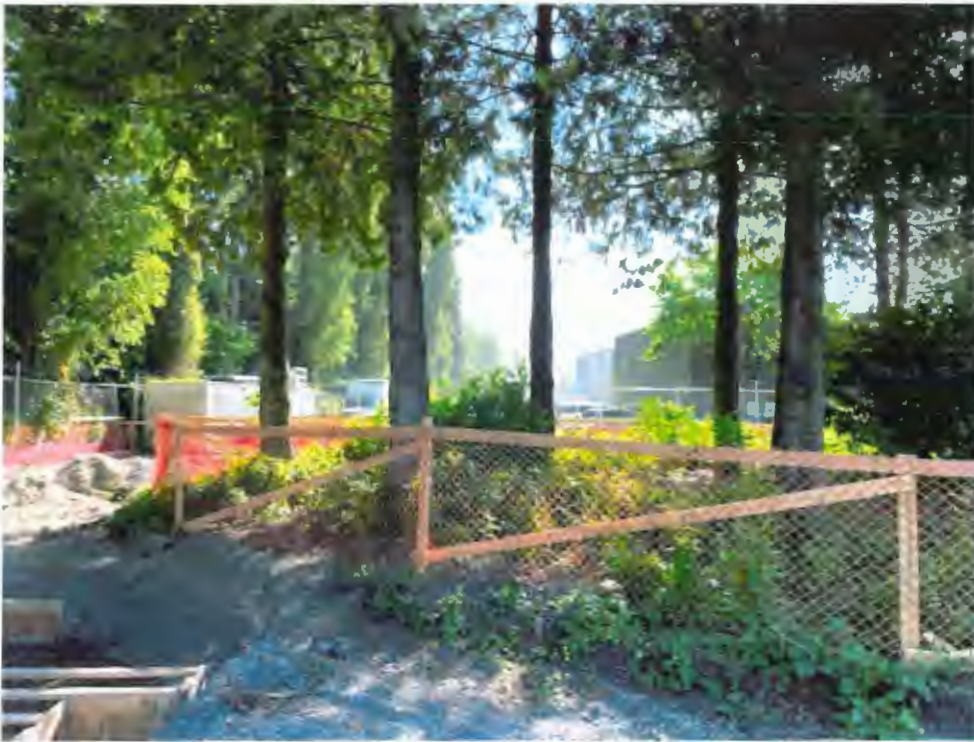
Photo 1: Southern ESA Fencing Protection looking northeast.
