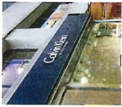
RECESSED OR INTEGRATED, INTERNALLY ILLUMINATED, OPAQUE ALUMINUM FACE WITH PUSH THROUGH ACRYLIC LETTERS.
