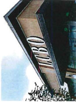
INDIVIDUAL METAL CHANNEL LETTERS ACRYLIC FACE - INTERNAL ILLUMINATION MOUNTED ON TOP OF CANOPY
