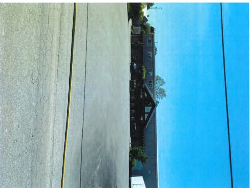
Figure 4. Current access to 12951 Blundell Rd (Parcel 1) via Sidaway Rd facing west. Access is approximately 11 m wide and leads directly to the processing facility and loading bay. Access is suitable for large trucks and trailers.
