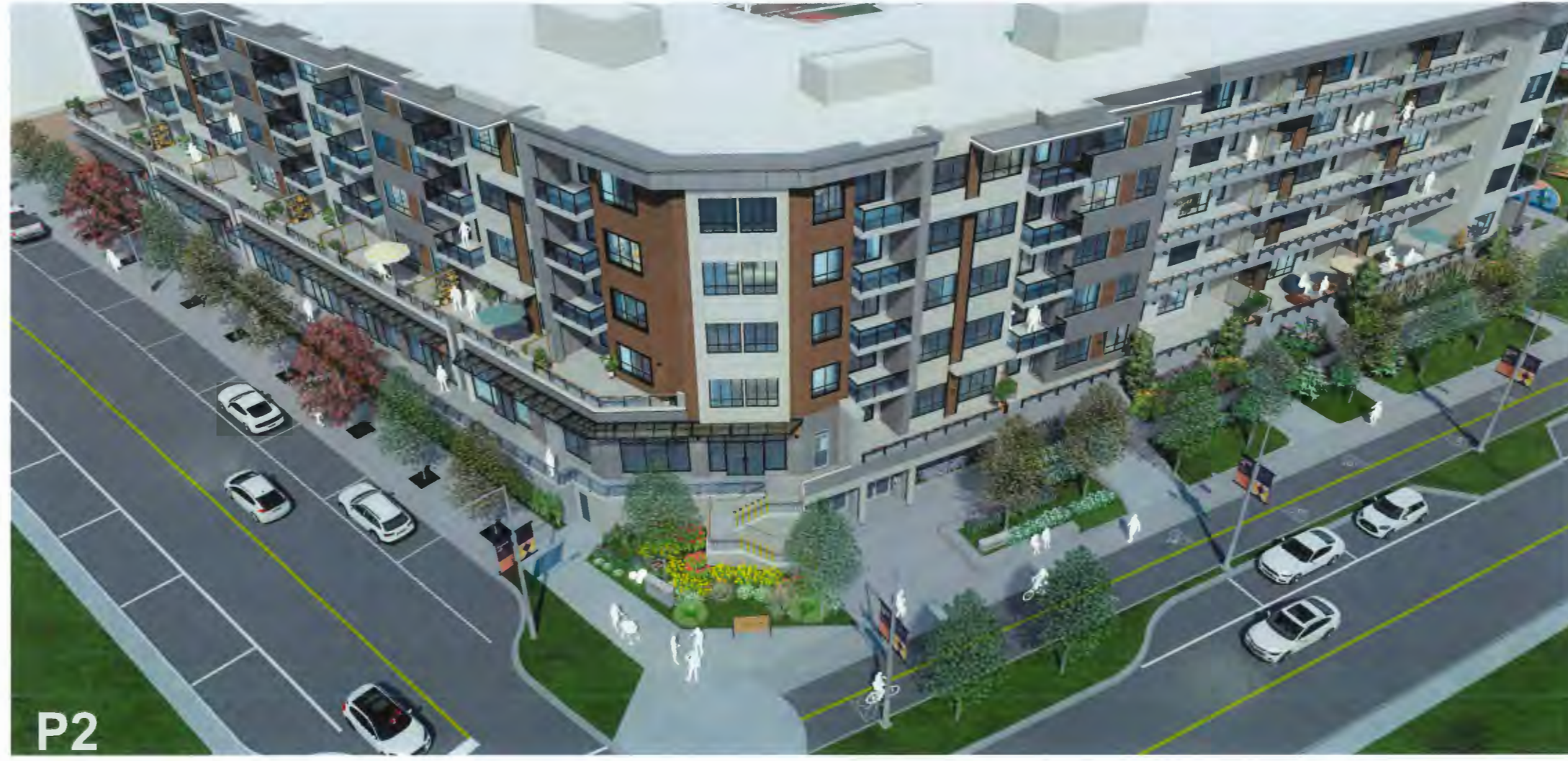
P2 building A - south-east corner view
