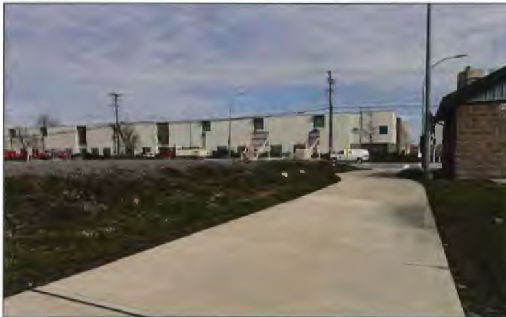
⑦ VIEW FROM BLUNDELL ROAD LOOKING EAST
