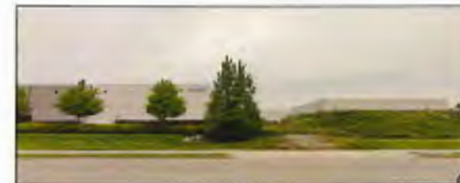
① VIEW LOOKING NORTH FROM BLUNDELL ROAD
