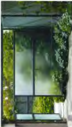
15 FROSTED GLASS PANEL WITH ALUMINUM FRAME
