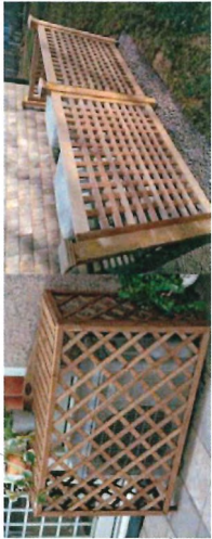
HEAT PUMP OUTDOOR UNIT WOOD SCREEN AT BACK YARD
