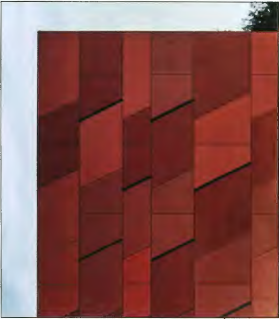
REFERENCE PICTURE - PARKADE ENTRY SOFFIT- FIBER CEMENT PANEL -SWISS PEARL LARGO CARAT - CORAL 7030, 7031, 7032
