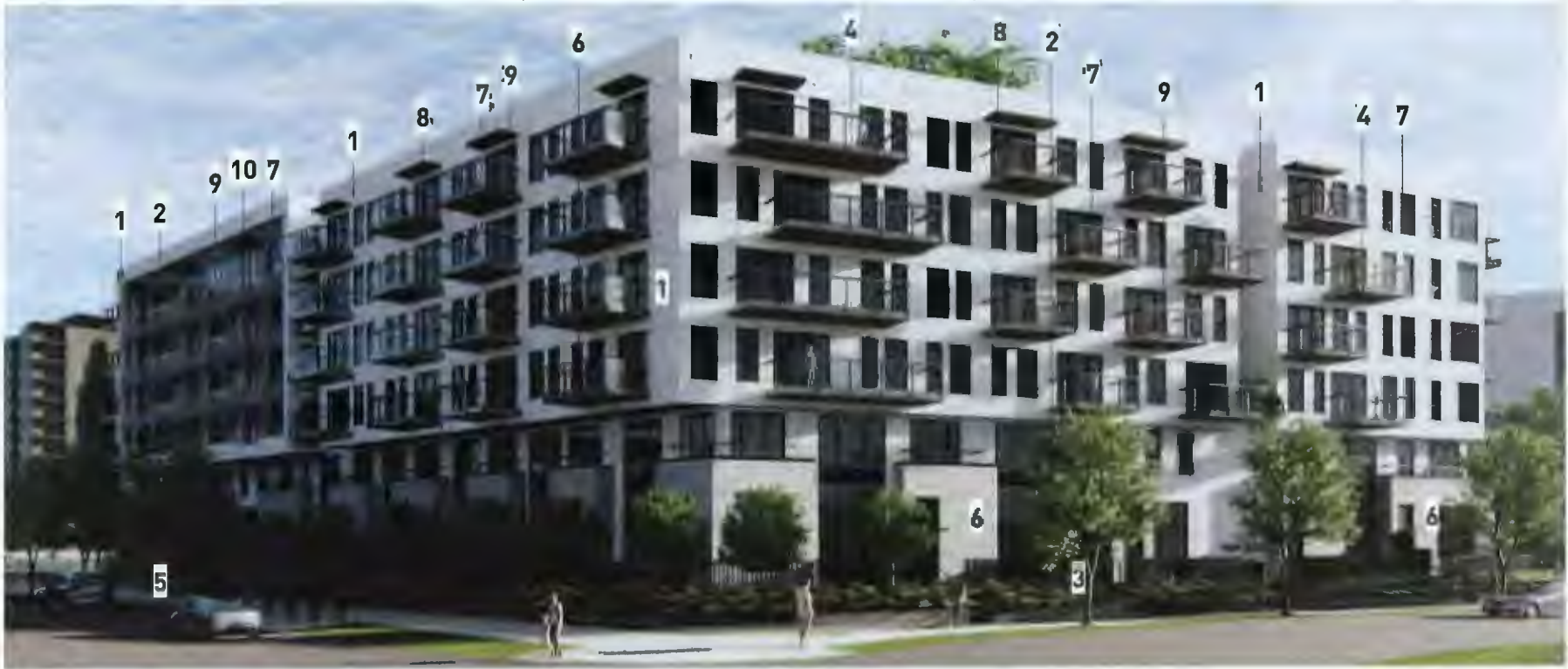
NORTH WEST VIEW
