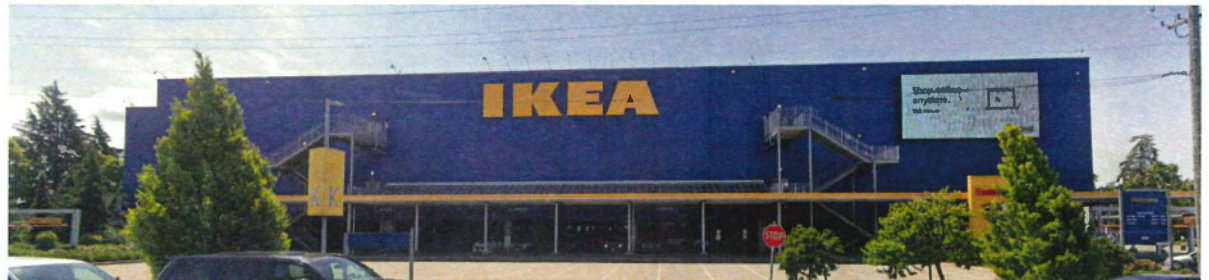
4 Existing North Exterior Parking View (Photos taken from Google Earth)
