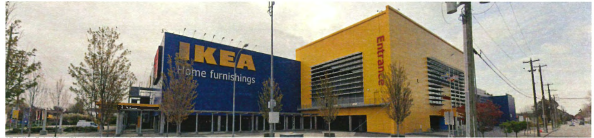
1 Existing Entry View (Photos taken from Google Earth)
