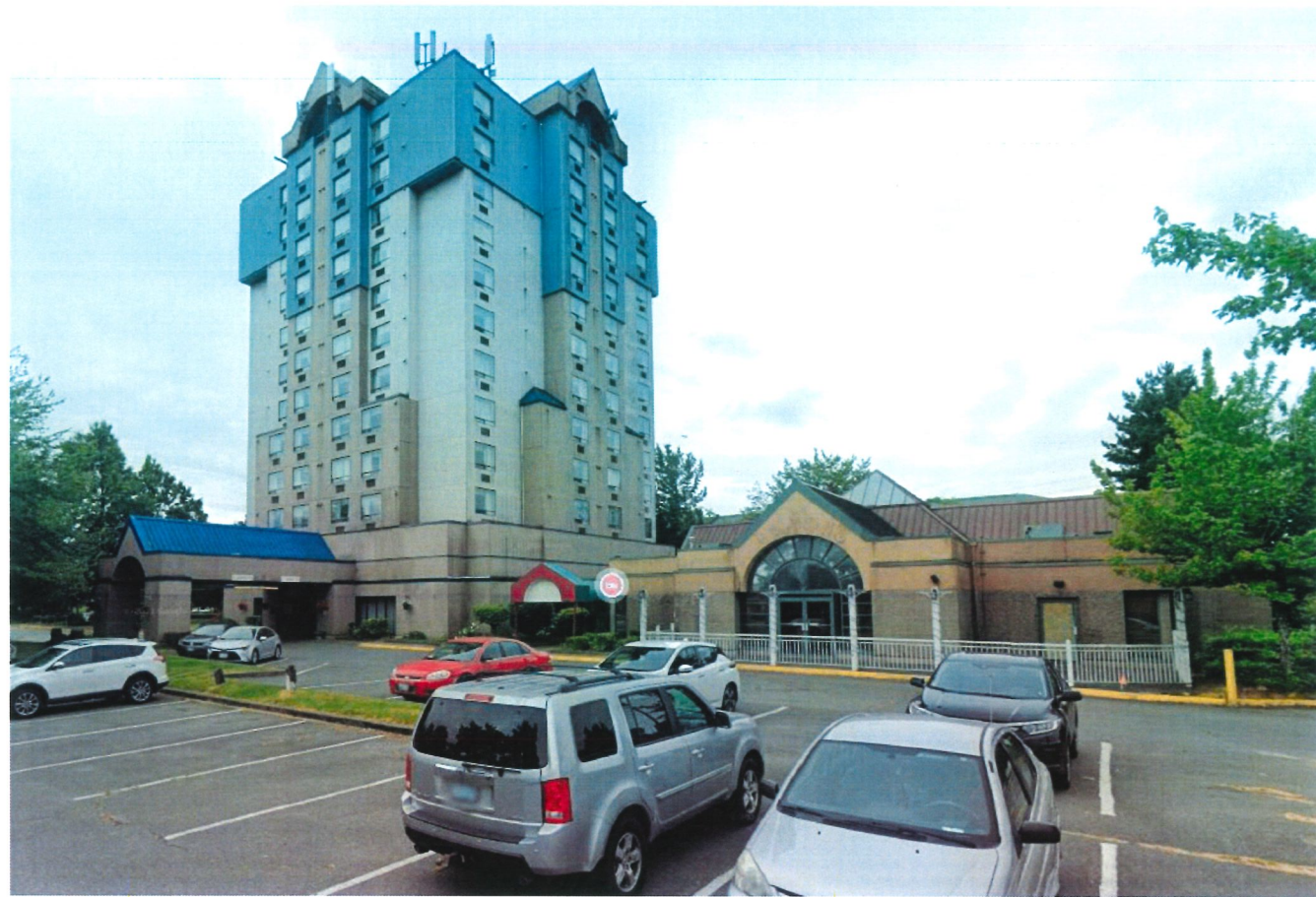
PICTURE OF EXISTING BUILDING
