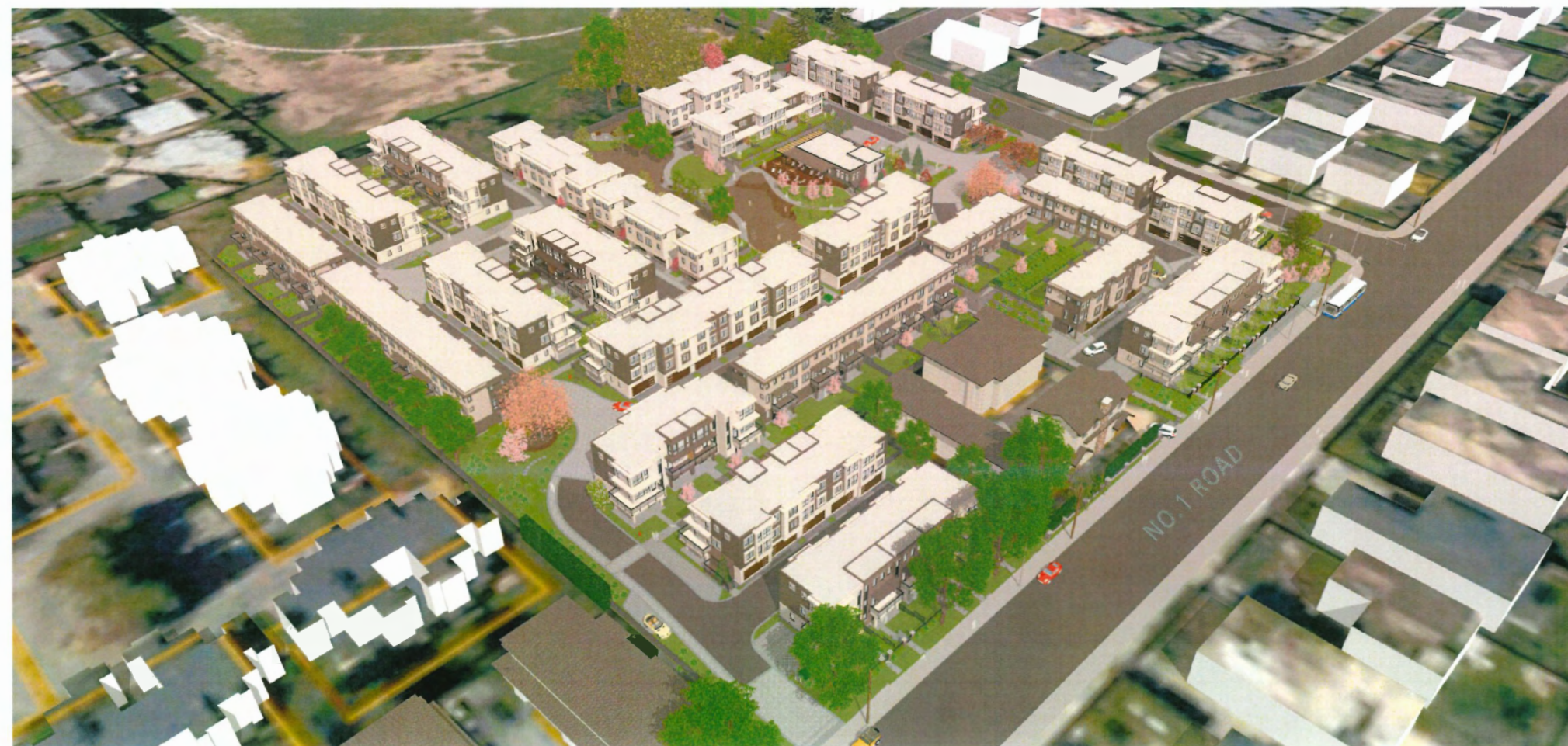
VIEW 2 AERIAL SE
