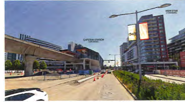
VIEW FROM NO. 3 ROAD LOOKING SOUTH
