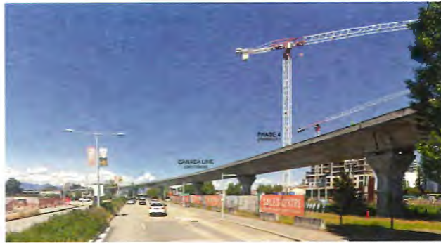
VIEW FROM NO. 3 ROAD LOOKING NORTH
