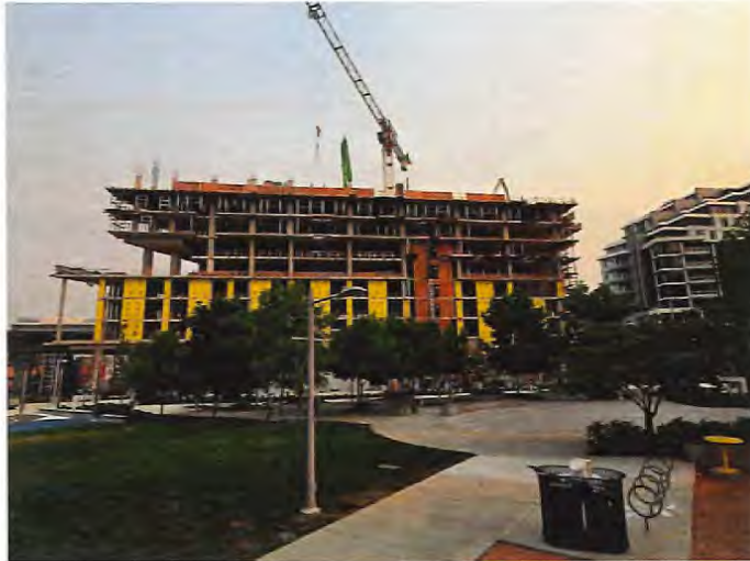
PHASE 4: BUILDING K September 5, 2025
