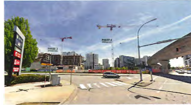
VIEW FROM NO. 3 ROAD & SEA ISLAND WAY
