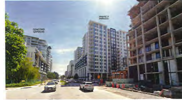
VIEW FROM NO. 3 ROAD LOOKING SOUTH
