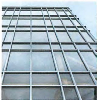
WW Window Wall Bypass Glazing System.
