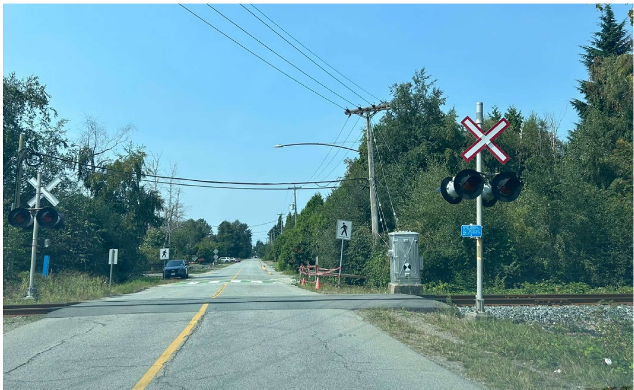
Current Conditions Looking Westbound
