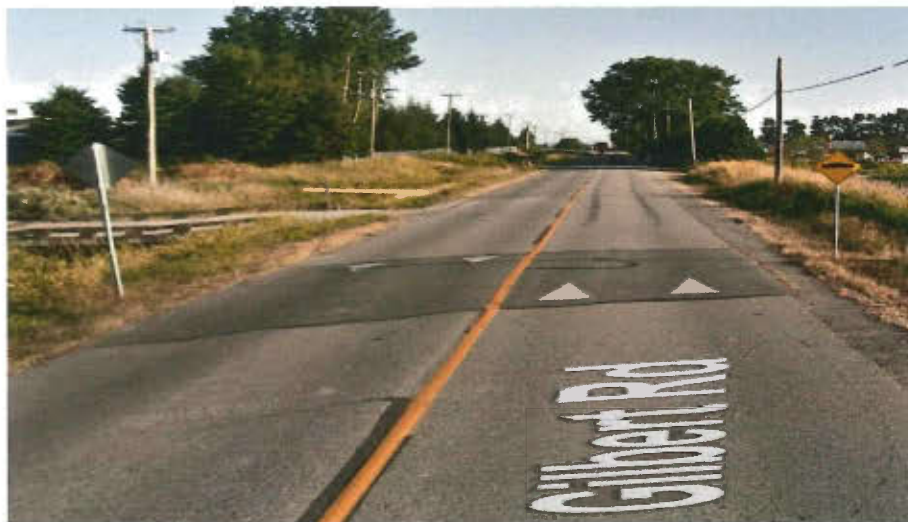
Example of Existing Speed Hump (as proposed) on Gilbert Road (south of Steveston Highway)
