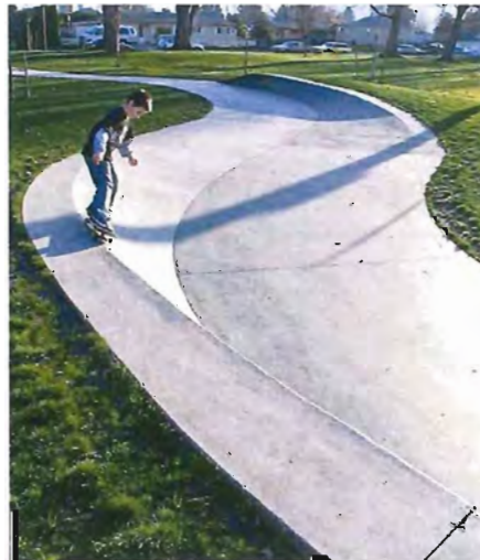
CONCRETE WAVE TO DIRECT DRAINAGE
