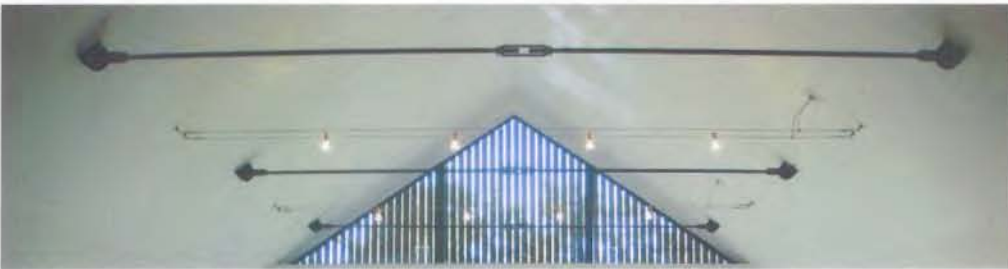
STEEL ROOF TIES TO EXTEND TO EXTERIOR GABLE END
