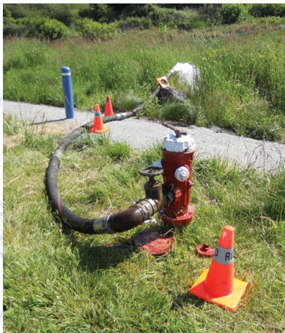
Water Services staff flushing the main line as part of the low flow flushing program
