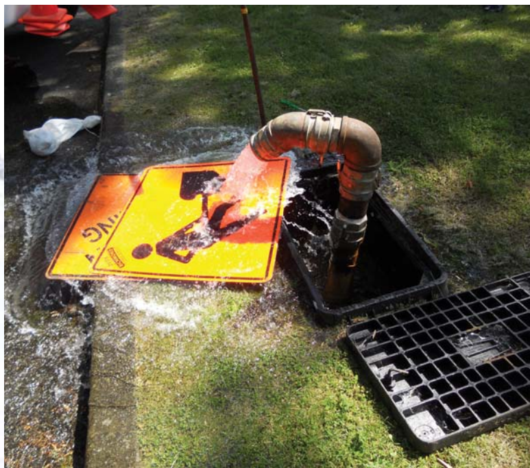
Water Services staff flushing the main line as part of the low flow flushing program
