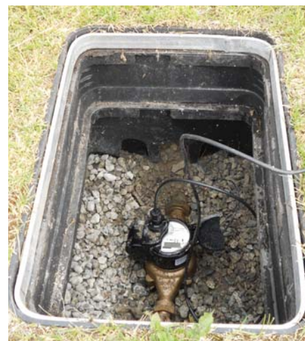
Installed water meter
