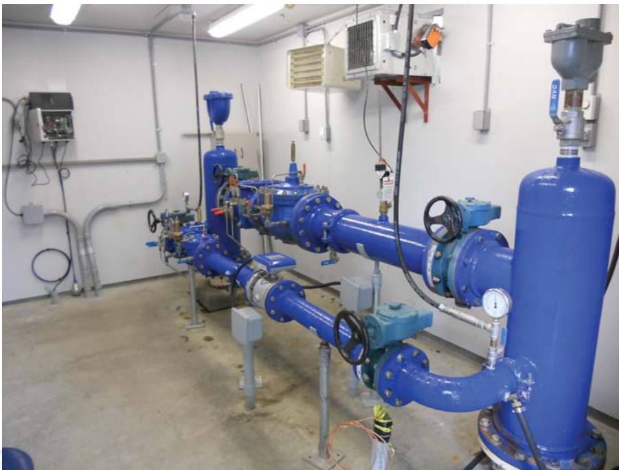
Inside the pressure-reducing valve station
