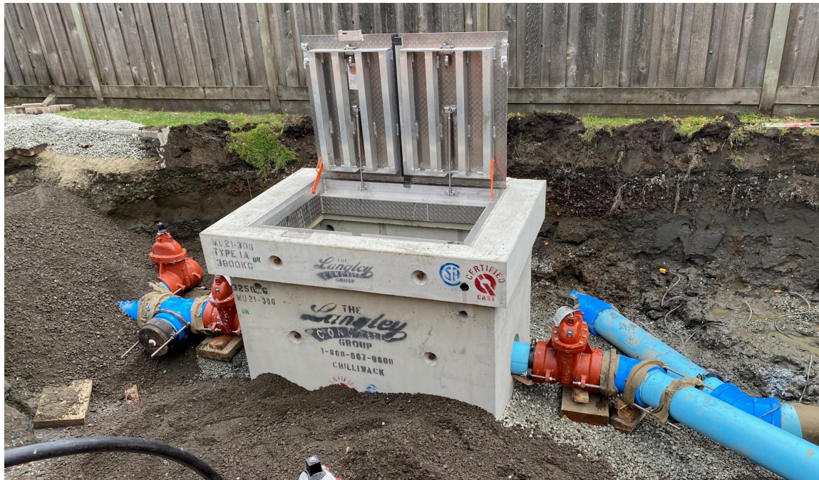
Multi-Family Water Meter Installation
