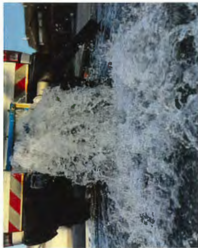
Flushing water using a truck-mounted water diffuser.
