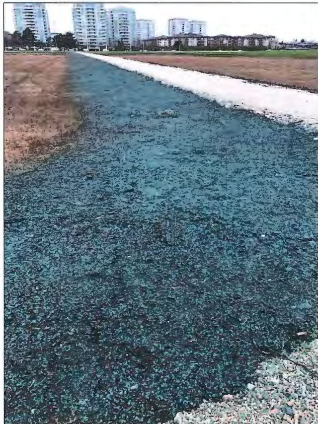
Above: Previously exposed soil after hydroseeding application.
