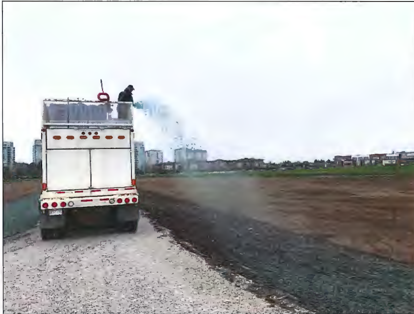
Above: Hydroseeding equipment applying native grass seed mixture to exposed soil slopes along farm access road.
