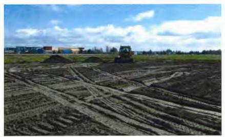
Figure 4 Soil being graded with dozer June 28, 2017
