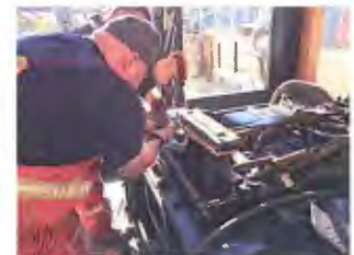
A new wooden plate was installed to balance the car when it is moved back into the trucks.
