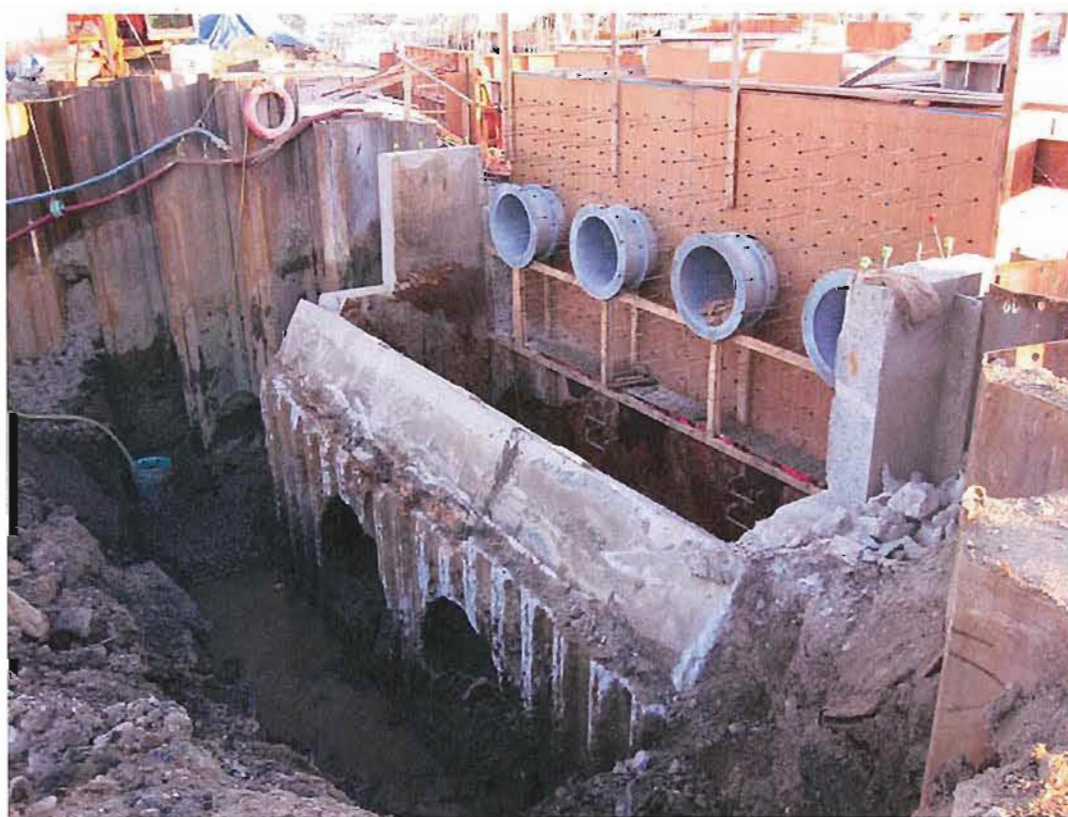
Flood Box Demolition/Construction
