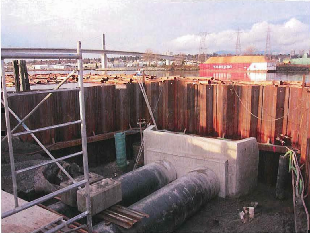
Gravity Discharge Pipes and Headwall
