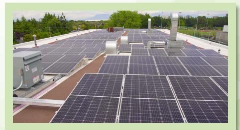
Brighouse Fire Hall No. 1. (6960 Gilbert Rd) is designed to withstand disasters and maintain operations post-event, and has a hybrid steel and mass timber roof. The facility optimized energy efficiency and achieved a LEED Gold certification. The facility was fitted with 136 solar panels that generate 60,000 kWh of electricity per year (equivalent of what 5 homes consume per year) and provide continuous power to the fire hall.
