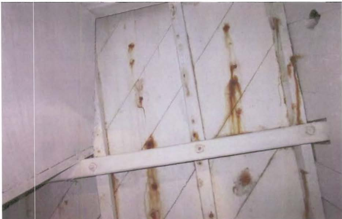
Photo #10 Detail of corroded fasteners inner planking
