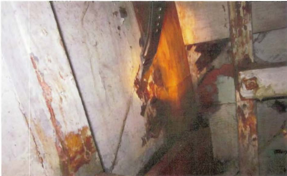
Photo #2 Deterioration of inner transom structure
