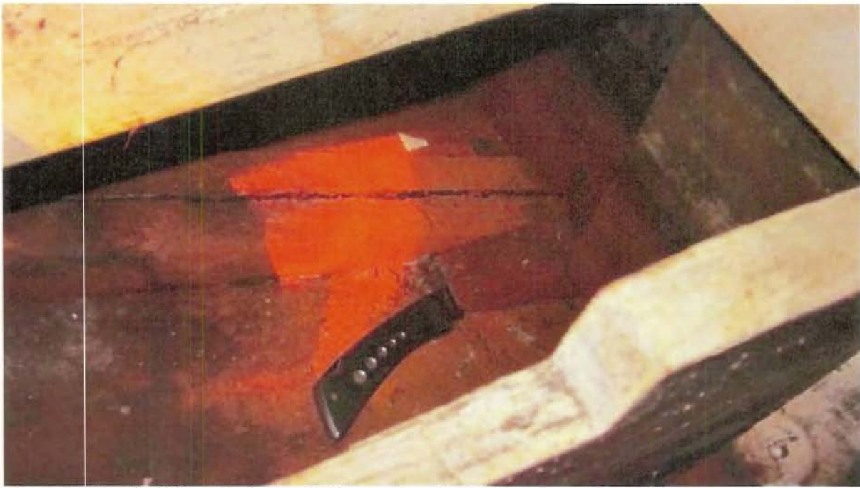
Photo #3 Detail of floor timber pulled away from hull
