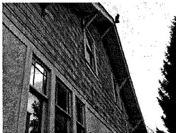
Shingle cladding at side gables
