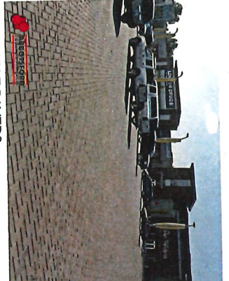
PERMEABLE PAVERS DRIVEWAY/AUTO COURT/ VISITOR PARKING PERMEABLE PAVERS ABBOTSFORD CONCRETE - AQUA PAVE COLOR: CHARCOAL
