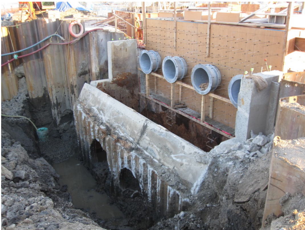
Flood Box Demolition/Construction
