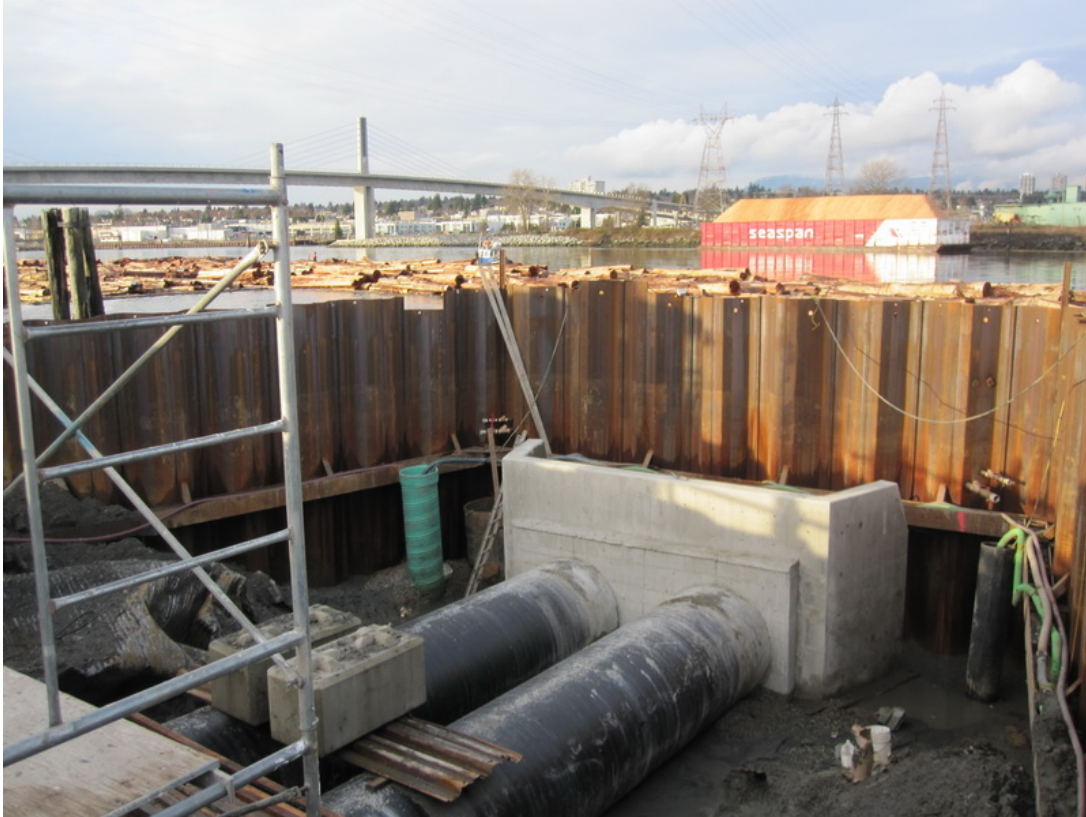
Gravity Discharge Pipes and Headwall
