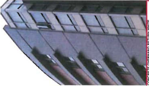
SPANDREL GLASS / WINDOW WALL
