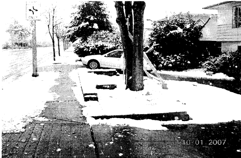
Photograph 2 shows the base of the two Maple trees (Trees # 5621, 5622). There is an approximate 0.4 meter grade difference between the sidewalk and the base of the trees.
