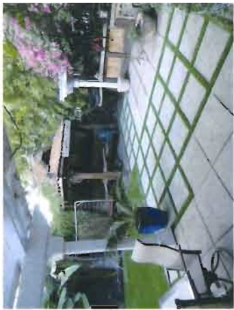
24X24 hyrapressed concrete pavers:
