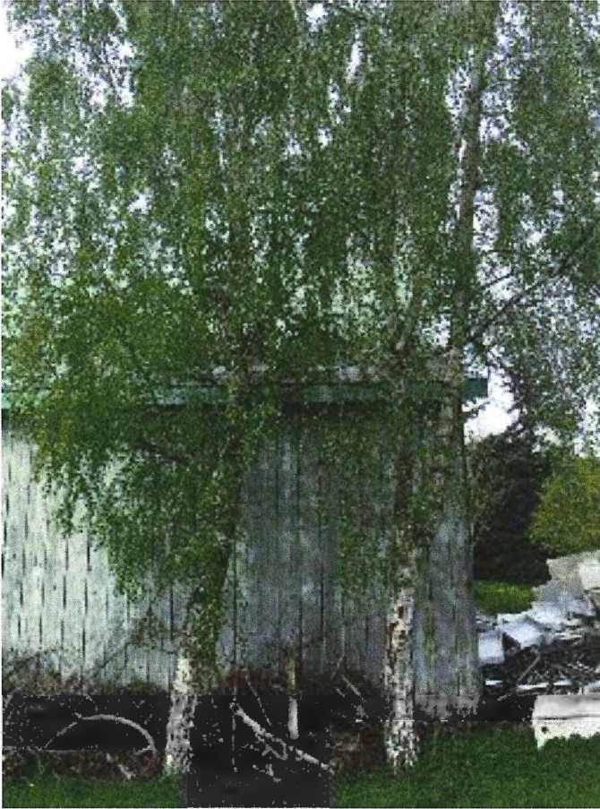
Figure 4 Two birch to be removed for shed demolition
