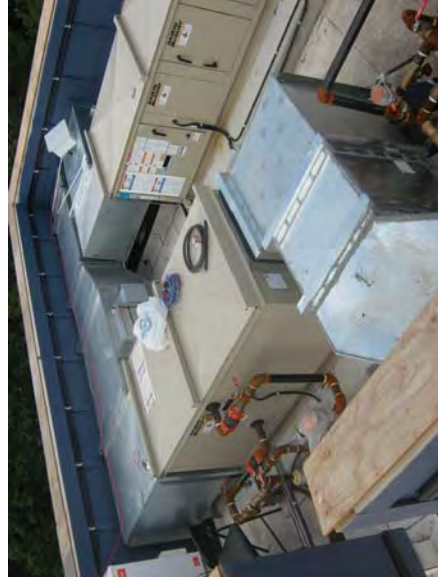
Mechanical and electrical equipment should be installed to facilitate ease of long-term maintenance. Avoid installing equipment in confined spaces or configurations, or in locations that have access problems. All City facilities must have a detailed Operations and Maintenance Plan detailed on the Consultants' Project Documents and on the Contractor's As-Built Documents, that demonstrates that all mechanical and electrical equipment can be accessed and maintained in a functional and workmanlike manner.
