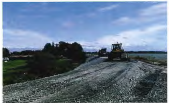
South dike upgrade from Gilbert Road to No. 3 Road Trail
