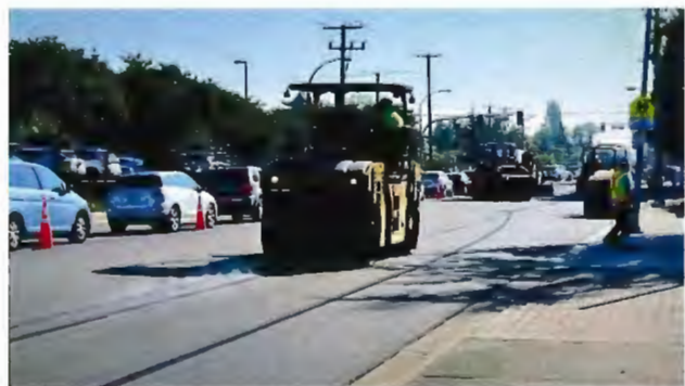
High Recycled Asphalt Pavement Project
