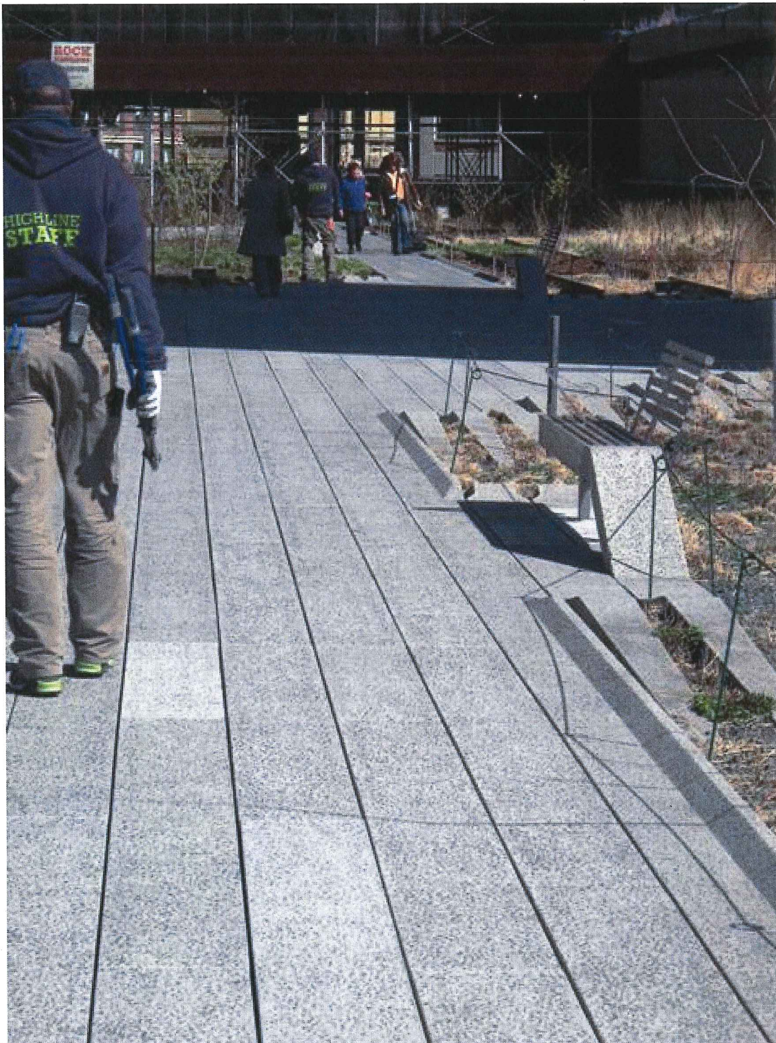
Concrete Textured to Appear as Wood Planks: Additional Examples
