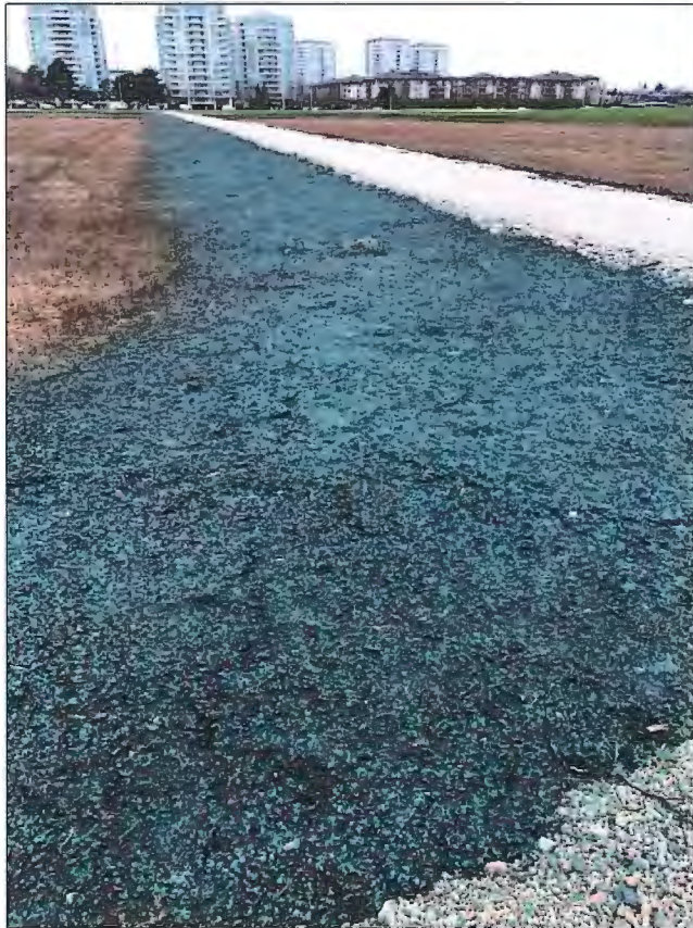
Above: Previously exposed soil after hydroseeding application.
