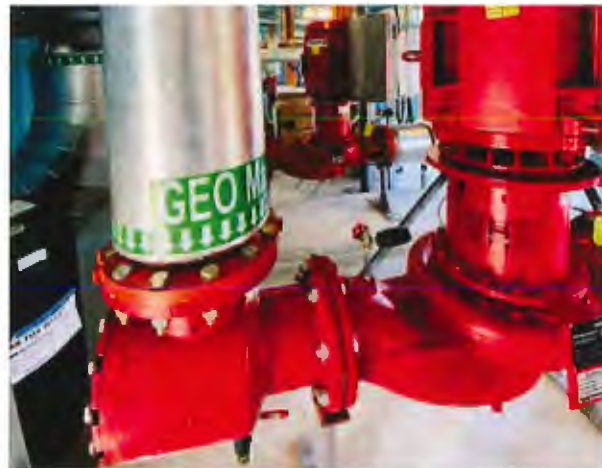
The Alexandra District Energy Utility distribution pumps disburse thermal energy through the underground pipe network.
