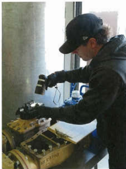
Water meter maintenance
