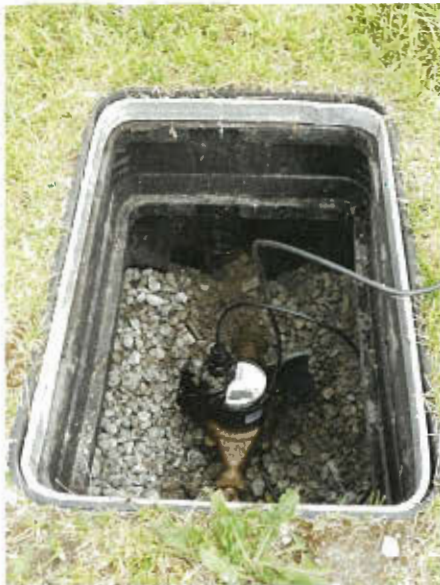
Residential water meter
