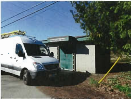
Shell Road and Bird Road PRV
