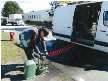
Regular maintenance on sampling site
