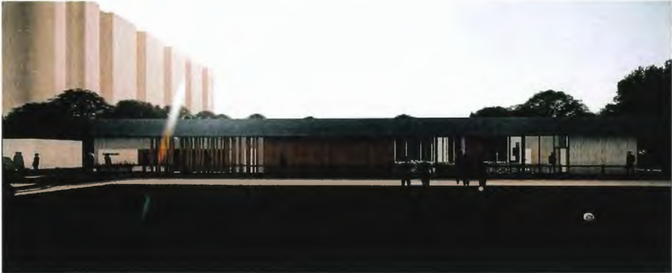
Figure 6. View from north green
